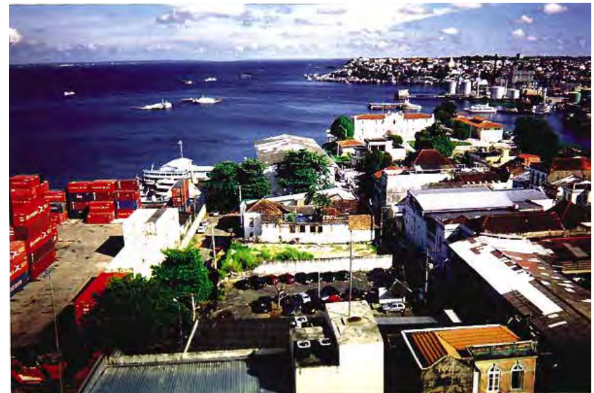
Overhead view of Project Area
